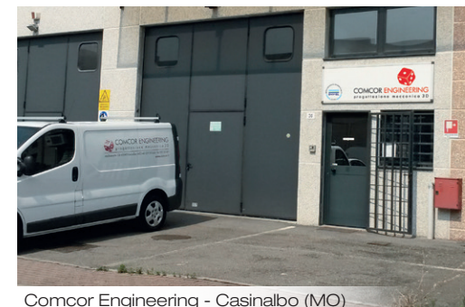
Comcor Engineering - Casinalbo (MO)
